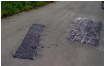
No the rain hasn't started falling in rectangles-evidence of pot-hole mending.
